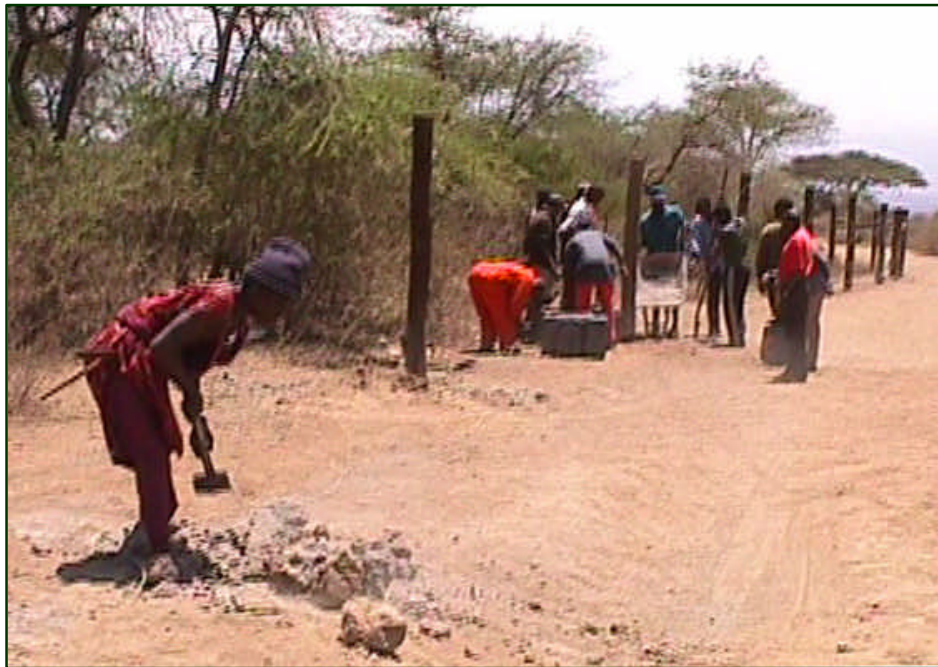
The KWS team of workers repairing the Kimana Fence, October 14
